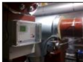
K47Flow 150 for heat quantity measurement application using PT100 sensors
